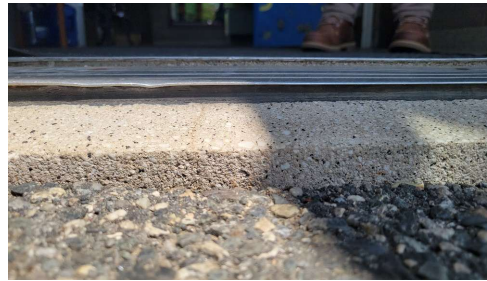
STEP AT MAIN ENTRANCE
