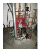
Heating for the building is provided by a single H.B. Smith, cast iron sectional hot water boiler. This boiler uses # 2 heating oil and has an output capacity of 174.8 MBH. Heating hot water is distributed via two fractional horsepower zone pumps to baseboard radiation located throughout the facility.
